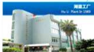
Huli Plant: 12,000 м 2
